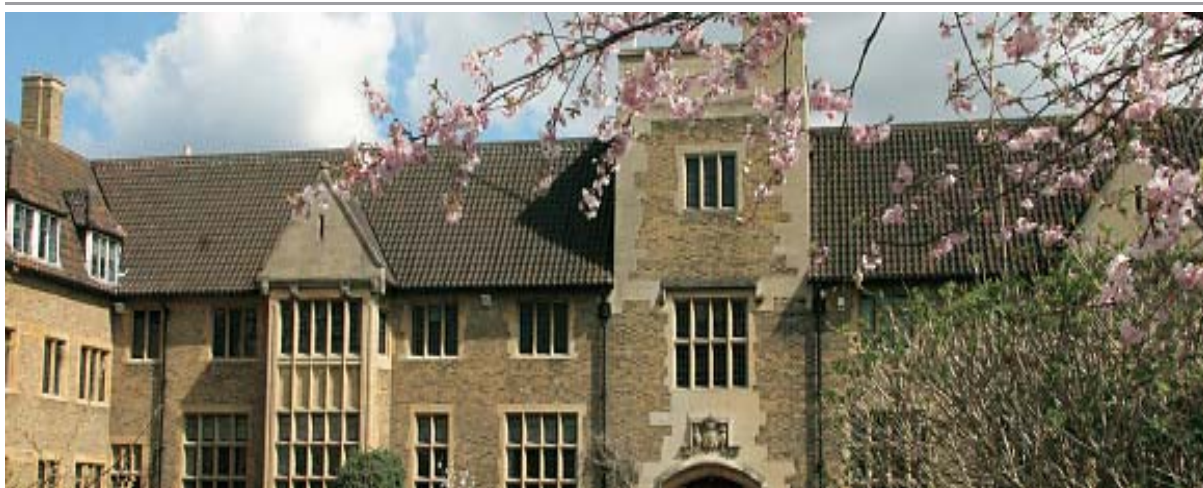
The magnificent Cheshunt College in Bateman Street, Cambridge, now the Province of Cambridgeshire Masonic Headquarters
